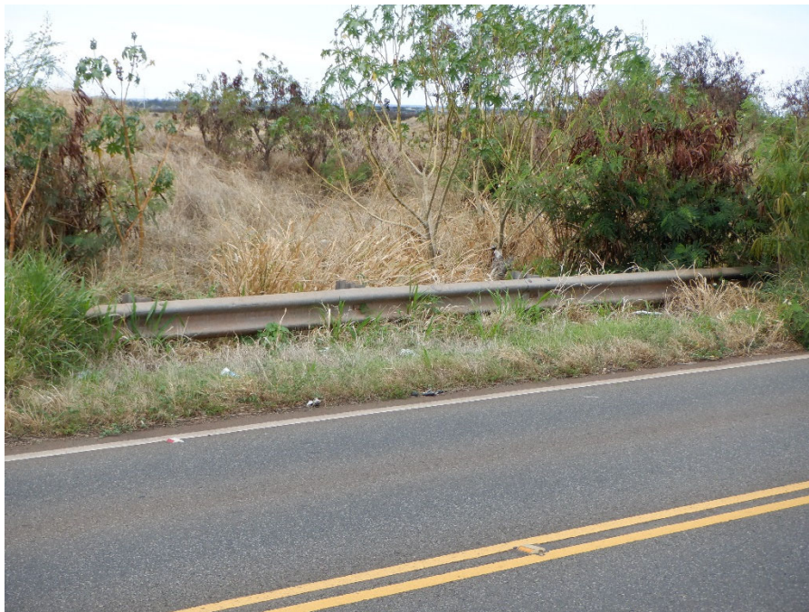
PHOTO 12 METAL GUARDRAIL ATTACHED TO DOWNSTREAM CONCRETE BRIDGE RAILING
