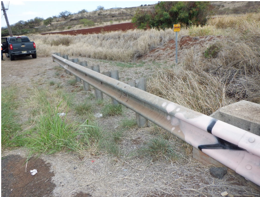
PHOTO 8 UPSTREAM WEST APPROACH GUARDRAIL
