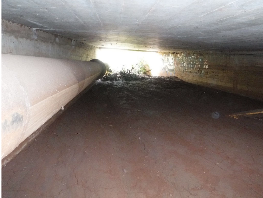
PHOTO 23 STREAM CHANNEL UNDER BRIDGE LOOKING UPSTREAM, WITH UTILITY PIPE ALONG ABUTMENT 2
