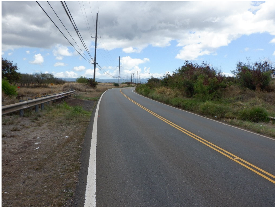
PHOTO 2 WEST APPROACH LOOKING EAST
