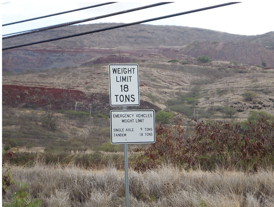
PHOTO 5 LOAD POSTING SIGNS ON FARRINGTON HIGHWAY AT EAST APPROACH TO BRIDGE
