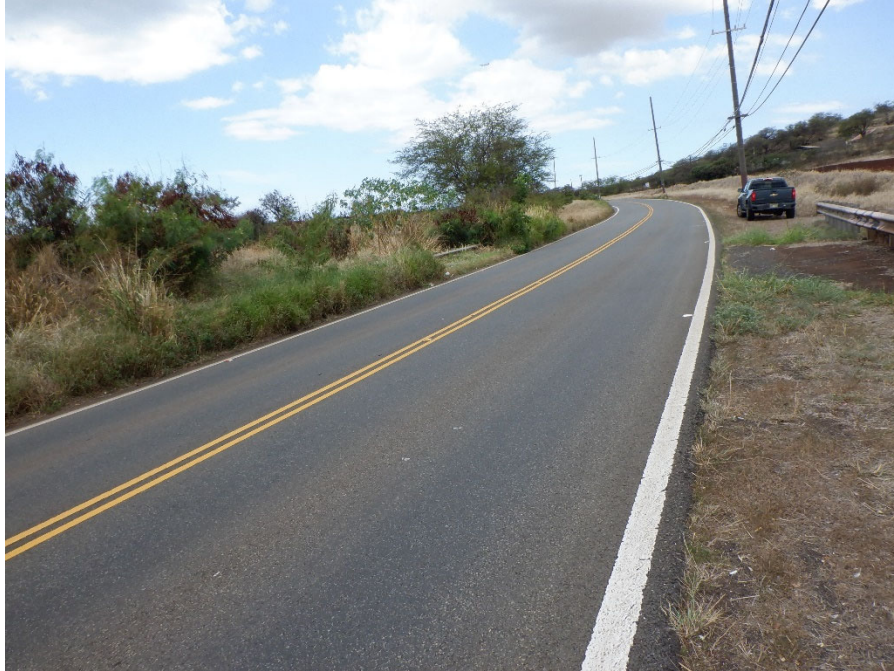
PHOTO 1 EAST APPROACH LOOKING WEST
