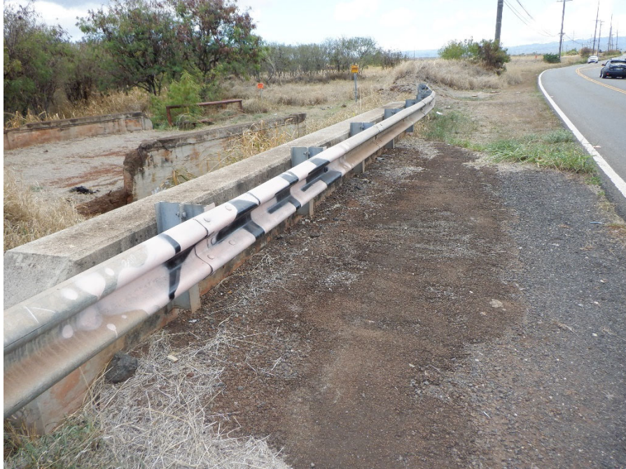
PHOTO 11 METAL GUARDRAIL ATTACHED TO UPSTREAM CONCRETE BRIDGE RAILING
